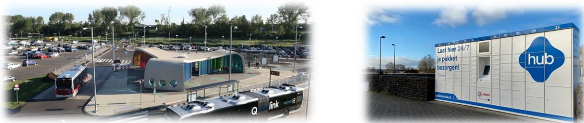
Figure 27: pictures of P+R and locker that was installed
